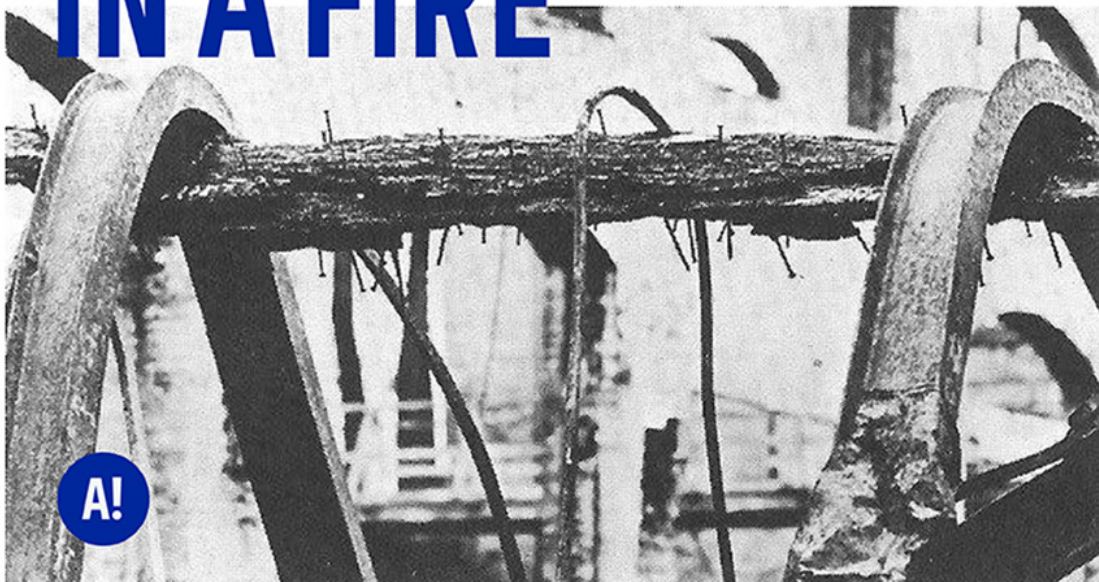
Fig 1. A wooden beam supporting two collapsed steel beams after the 1906 San Francisco fire
